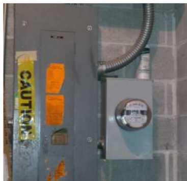
Figure E6: Sub-meter for Charles Schwab
