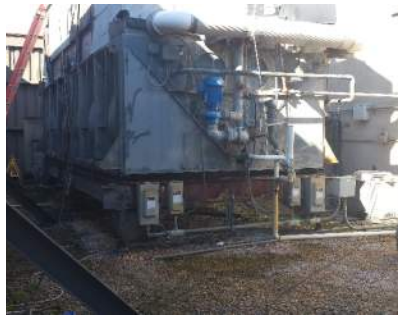
Figure M1: The existing Cooling Tower
