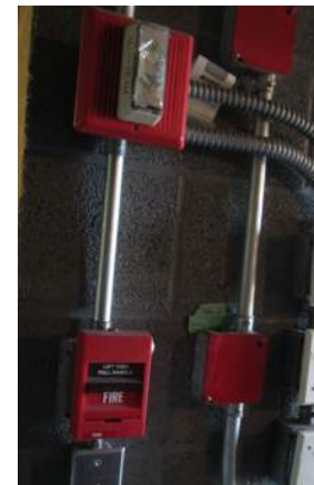
Figure E22: Typ. Fire Alarm Devices
