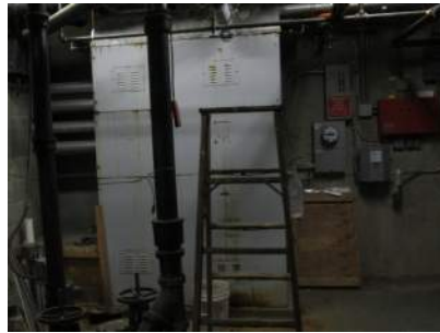
Figure E2: Existing Utility Pullbox
