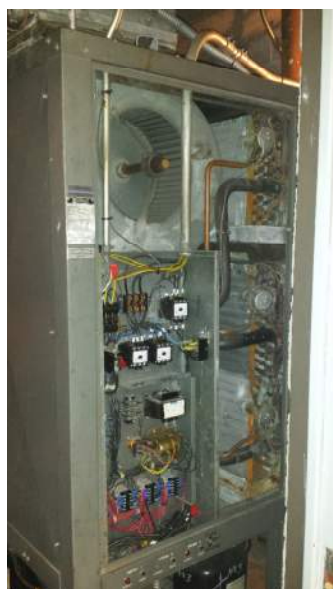
Figure M5: Existing Central AHU
