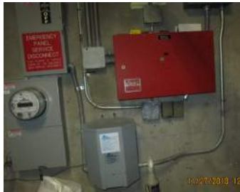
Figure E18: Emergency Light from Service
