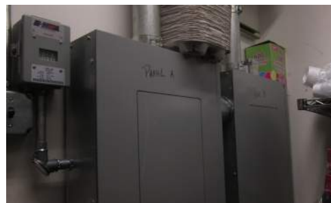
Figure E7: Sub-meter for Deli
